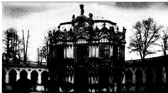
Pavilion of the Zwinger palace, Dresden, Germany, 1709, by Matthäus Pöppelmann (1662-1736)
