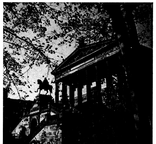
The National gallery built in the form of a Corinthian temple, 1866-76, by H. J. Strack
