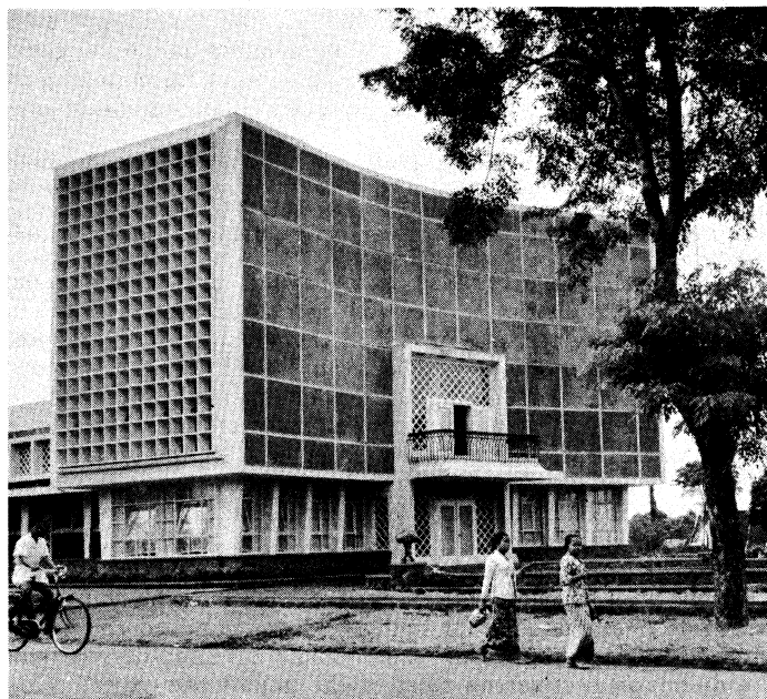
WAAGENAAR-PIX FROM PUBLIX MATHEMATICS AND PHYSICS BUILDING OF THE UNIVERSITY OF INDONESIA AT BANDUNG
